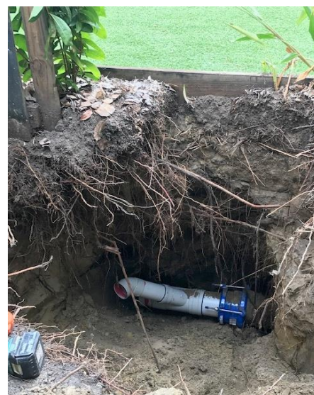
Images: House connection branch lines repaired and restored to original state in Port Douglas area.
