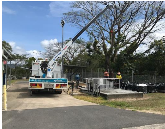
Image: Contractor's servicing wastewater pumps within Douglas Shire
