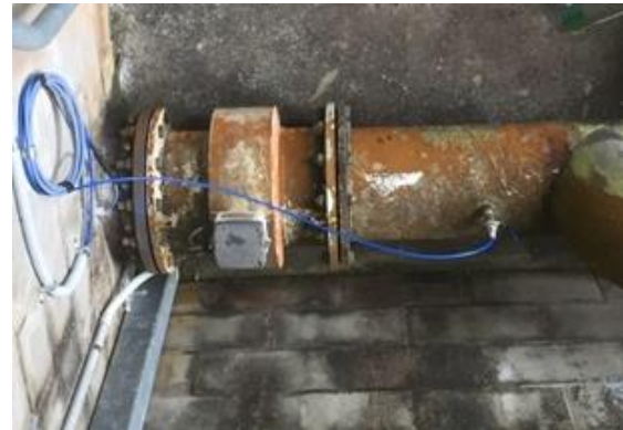
Images: Water Quality team installing the communications of the chlorine/pH analyser
