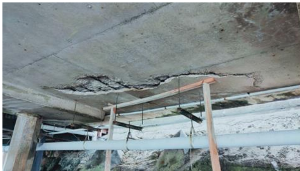
Images: Delaminated / spalled concrete before and after removal
