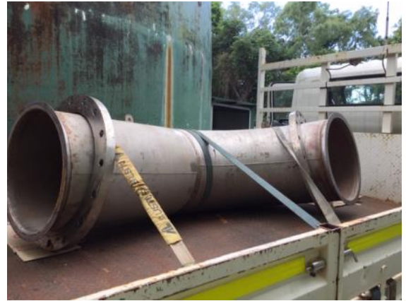
Images: Inspecting Dawsons Engineering proposed repair works on raw water main pipework
