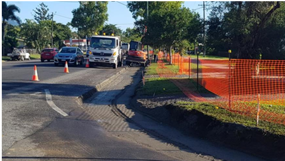
Image: Alchera Drive removing the old kerb and channel and prepping the base
