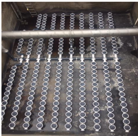
Images: Digester 1 & 2 (diffuser) aeration system replacement at Port Douglas WWTP
