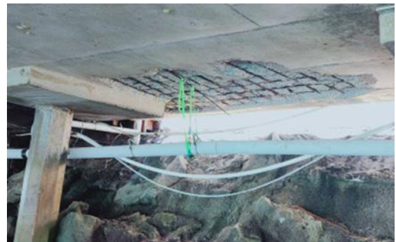
Images: Delaminated / spalled concrete before and after removal
