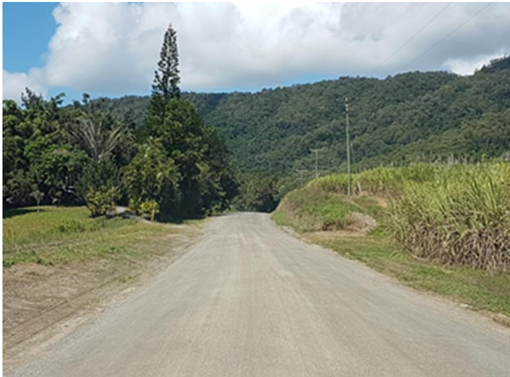
Image: Gravel resheet completed on Upper Cassowary Road
