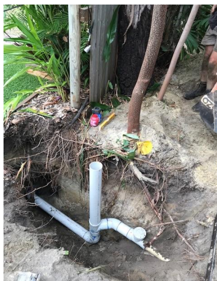
Images: House connection branch lines repaired and restored to original state in Port Douglas area.
