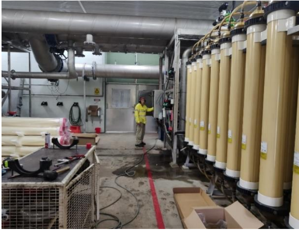
Images: UF cartridges installed at Mossman and Daintree Water Treatment Plants
