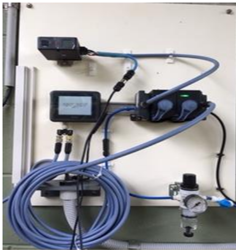
Images: Water Quality team installing the communications of the chlorine/pH analyser
