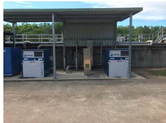
Images: Digester blowers and SBR aeration blowers installed at Port Douglas Wastewater Treatment Plant
