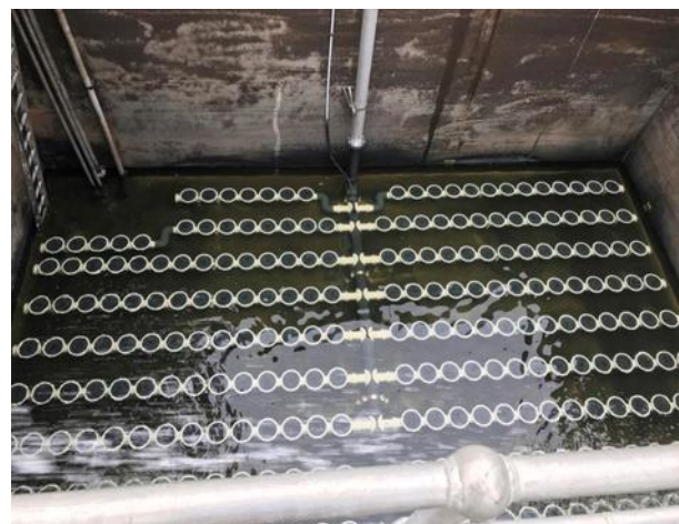
Images: Digester 1 & 2 (diffuser) aeration system replacement at Port Douglas WWTP
