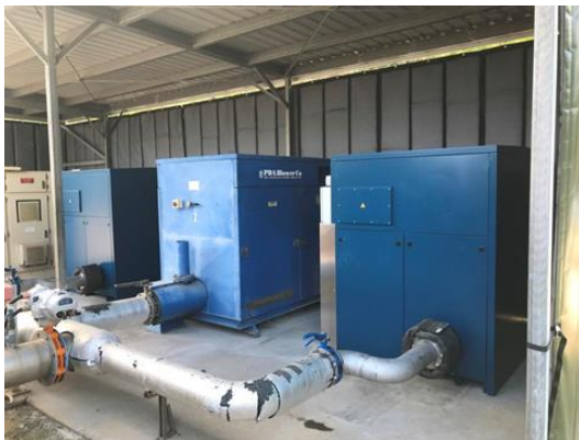
Images: Digester blowers and SBR aeration blowers installed at Port Douglas Wastewater Treatment Plant
