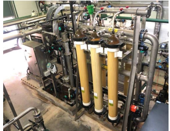
Images: UF cartridges installed at Mossman and Daintree Water Treatment Plants
