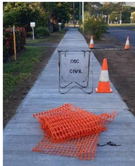
Images: Hart Street footpath renewal and upgraded to a 2.0m wide new concrete footpath Ordinary Council Meeting - 19 October 2021
