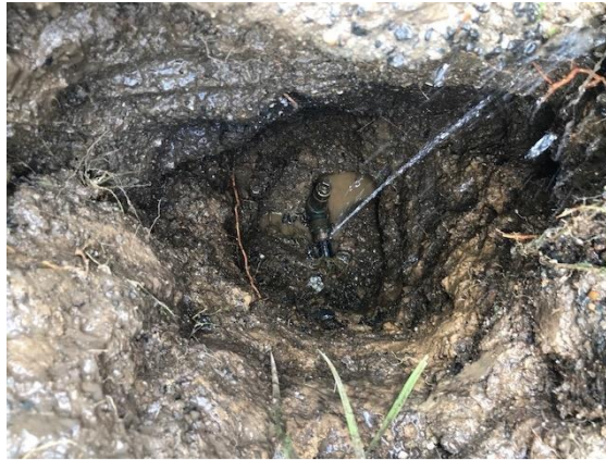
Image: Water leak which had a dual metered property connection
