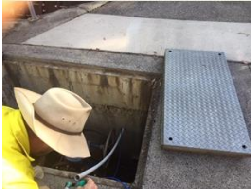
Images: Water Quality team installing the communications of the chlorine/pH analyser
