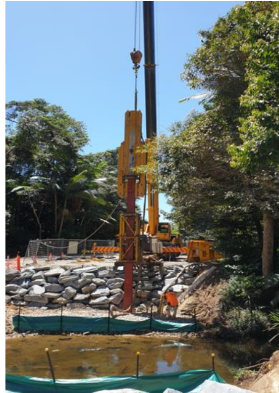
Images: Contractor installing Piles at Anich's Bridge
