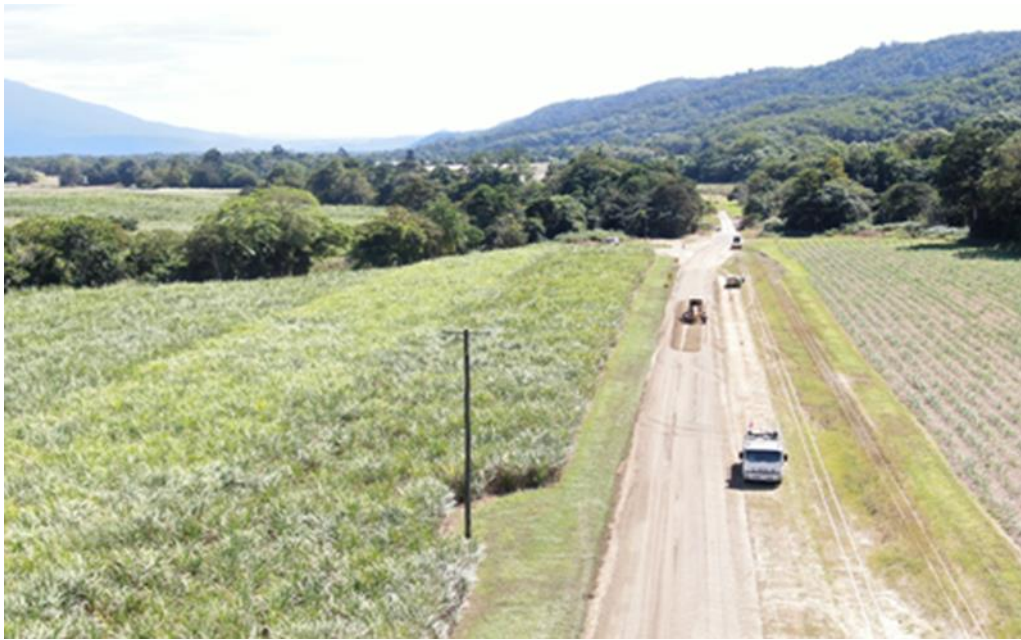
Image: Upper Cassowary Road receiving 70mm gravel resheet and drainage upgrade
