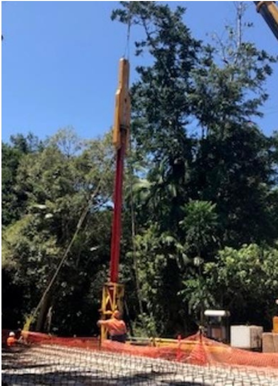
Images: Contractor installing Piles at Anich's Bridge
