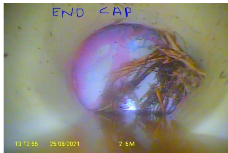
Image: Tree roots infiltrating a sewer main pipe
