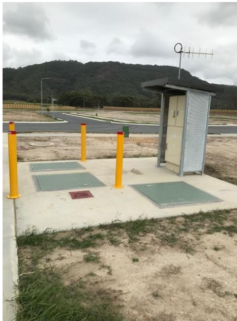
Images: new sewer pump station and council sewer reticulation in Craigie subdivision
