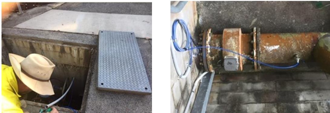
Image: Water Quality team installing the communications of the chlorine/pH analyser
