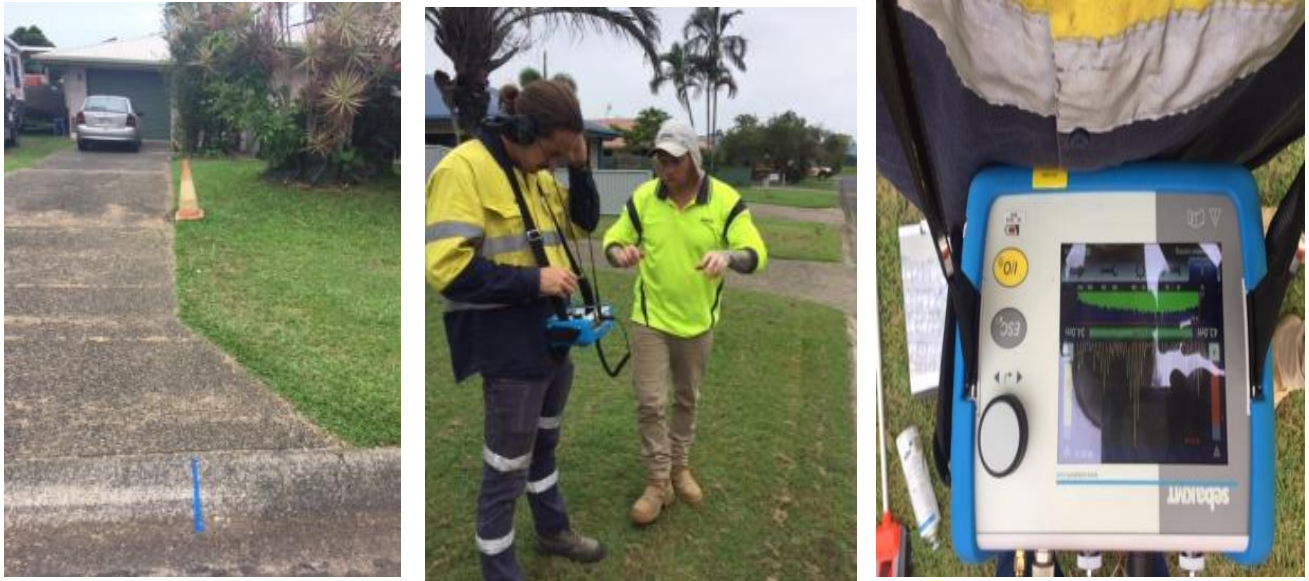
Water reticulation team locating water leaks
