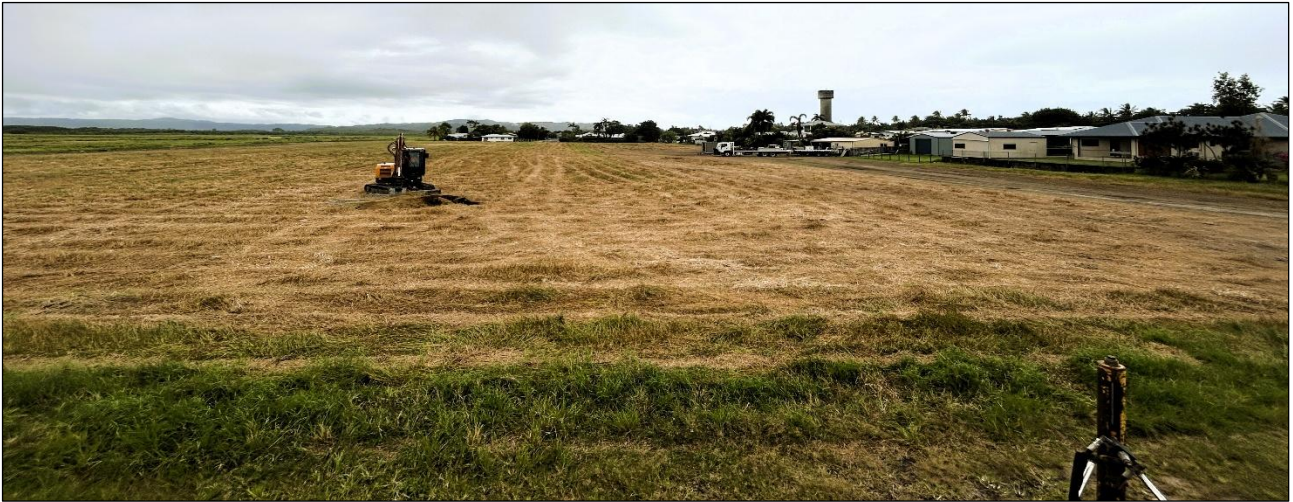
Figure 1: Looking north across site from the southern boundary; excavator at Pit 1.
