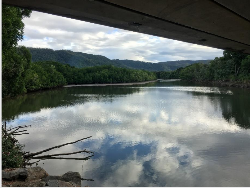
Upstream view of current bridge over Mowbray River
