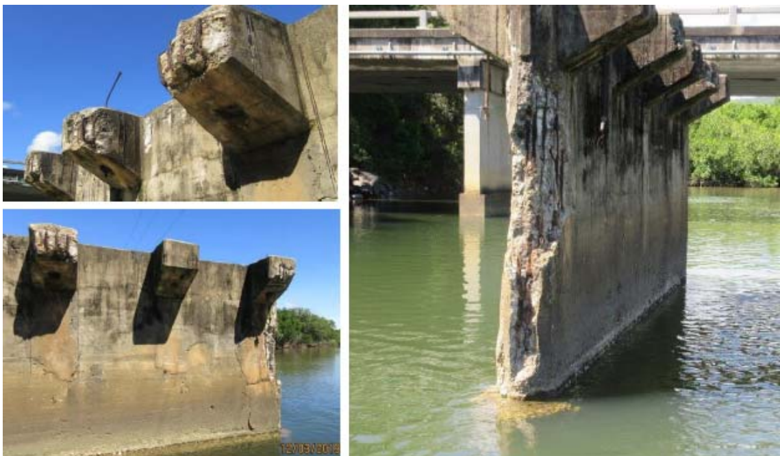
Plate 3-7 Photos showing defects of the existing piers
