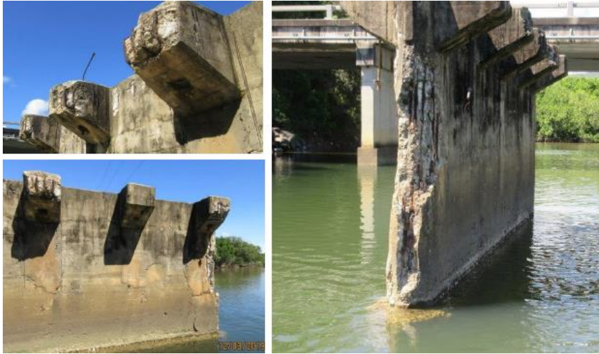
Figure 3-3 Photos showing defects of the existing piers
