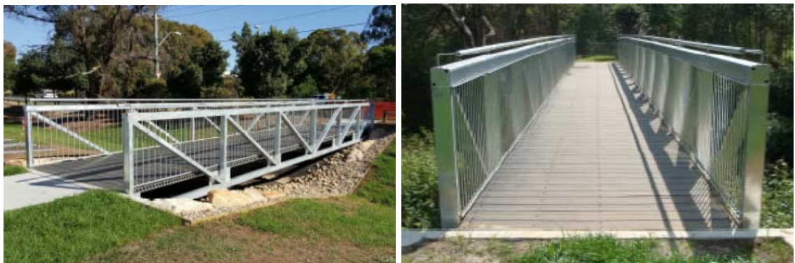
Plate 3-1 Example of single span bridges for B38 and B39
