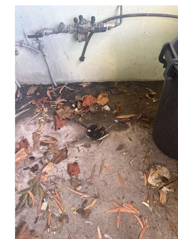
EXISTING WASHDOWN DRAIN
