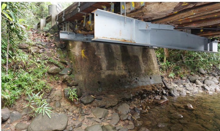
Northern abutments of Noah Creek bridge at low tide. Both banks on either side are very steep, the eastern side being more so
