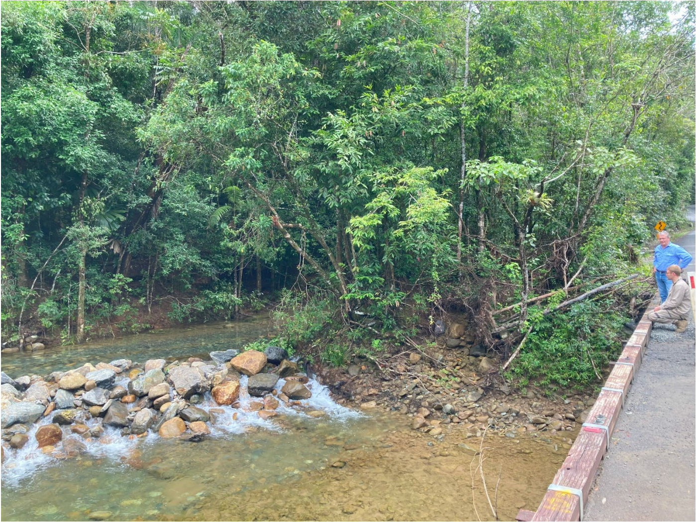
Figure 6. Noah Creek bridge impact area, north-west bank which is marked for clearing.
