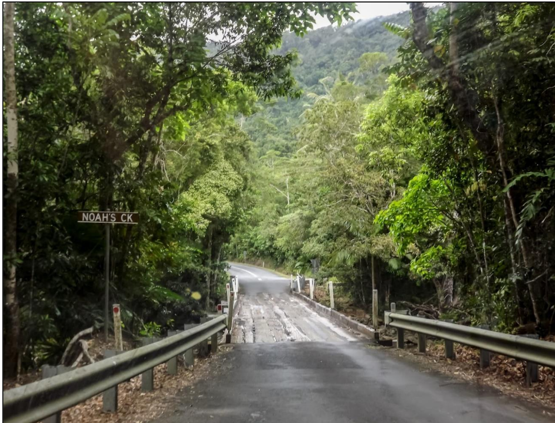
Figure 2 Noahs Creek Bridge Prior to Cyclone Jasper
