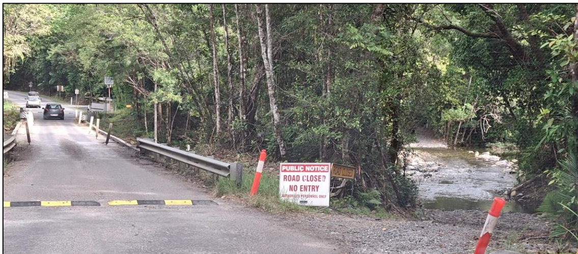
Figure 3 Noahs Creek Bridge and Existing Temporary Bypass - View Looking South
