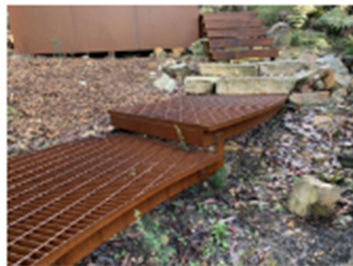
Alternative pathway material choice (steel over hardwood, also allows for some light permeation).
