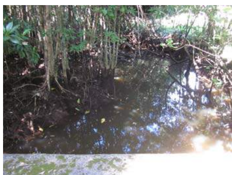
Upstream of Lutra Bridge
