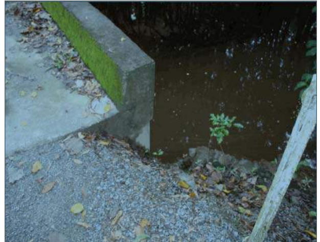
Approach to Lutra Bridge eroding
