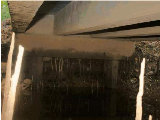
Erosion exposing the abutment under Lutra Bridge
