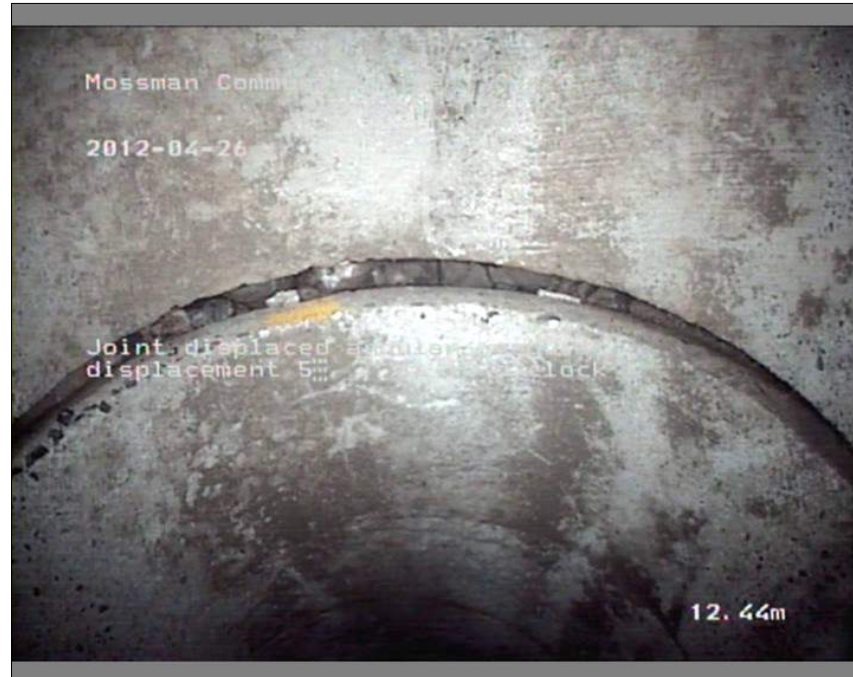
Photo: 7_8_30_A.JPG 12.44m, Joint displaced angular, angular displacement 5° , at 12 o'clock
