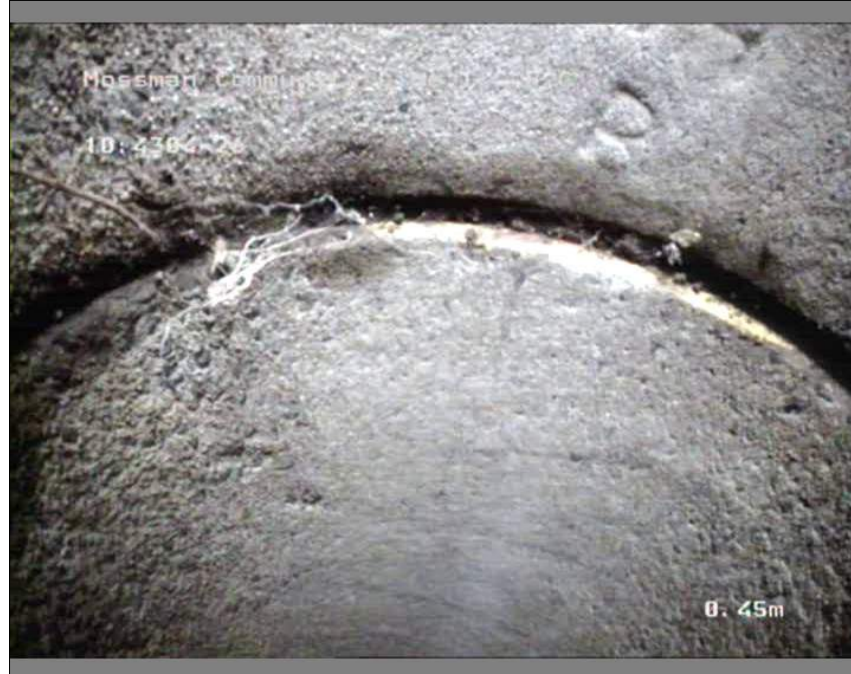
Photo: 7_8_28_A.JPG 0.45m, Joint displaced longitudinally, longitudinal displacement 10-20mm
