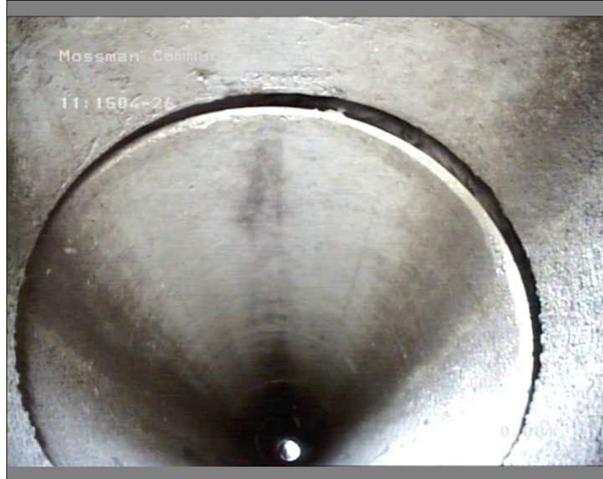
Photo: 9_10_40_A.JPG 0m, Joint displaced angular, angular displacement 10° , at 2 o'clock
