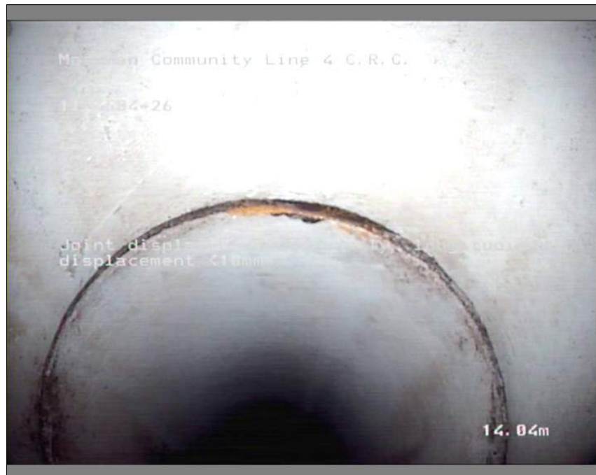
Photo: 11_12_55_A.JPG 14.04m, Joint displaced longitudinally, longitudinal displacement <10mm
