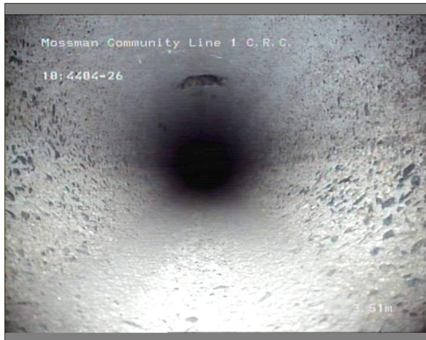
Photo: 7_8_29_A.JPG 3.51m, Some coarse aggregate is visible , Obstruction: <5% , from 12 to 12 o'clock
