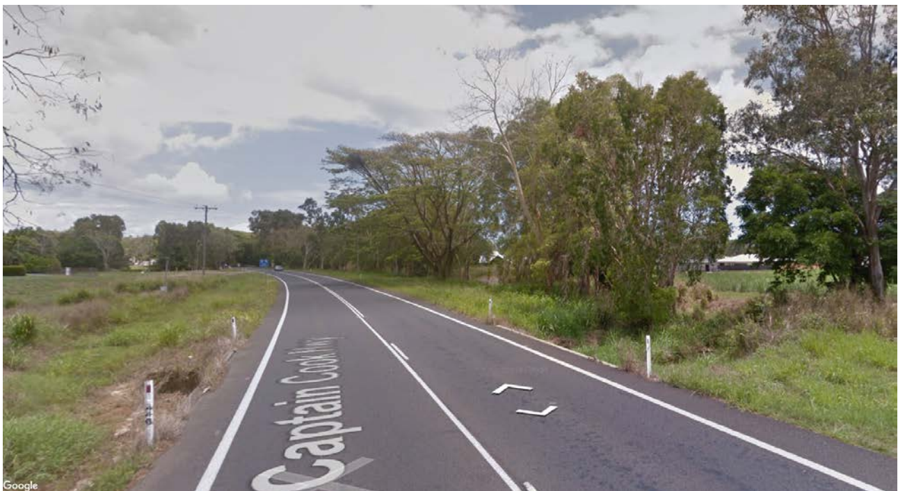
Figure 2: View north along the Captain Cook Highway – Culvert Crossing (source Nearmap Dec 2018)
