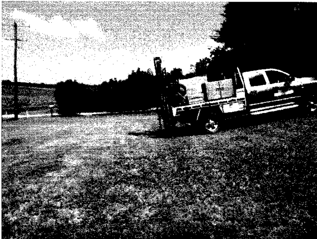
BH1 being drilled at 8 DeMeio Drive, Lower Daintree
