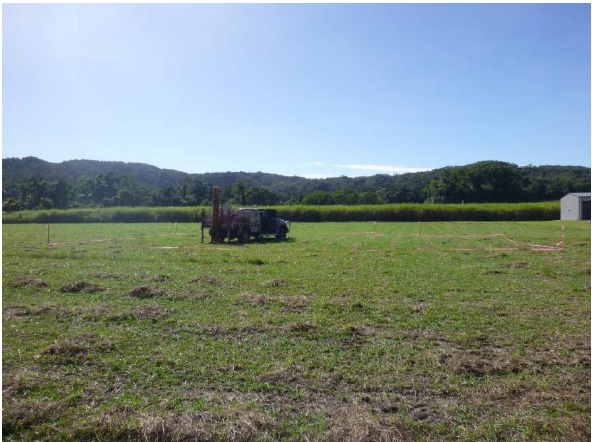
BH1 being drilled at Lot 14 Bamboo Creek Road, Miallo
