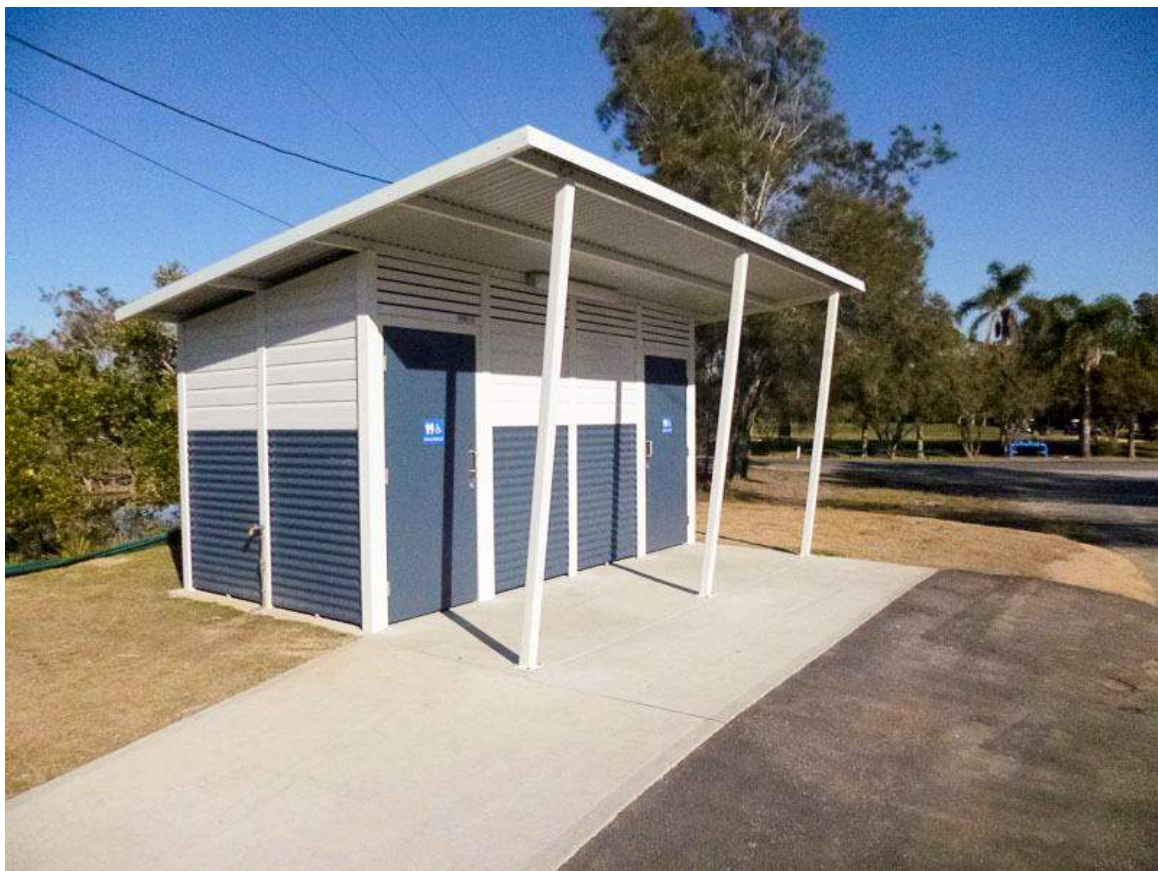
Yarra-2 Toilet Building
