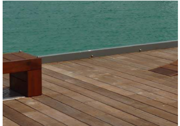
Natural Timber Boardwalk, Port Coogee, WA.
