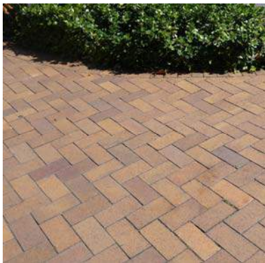
Paving, Port Douglas.
