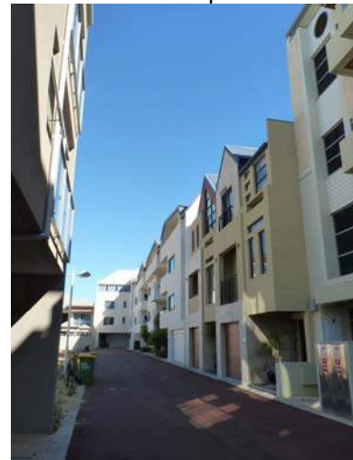
Access lanes to waterfront buildings – no landscaping.
