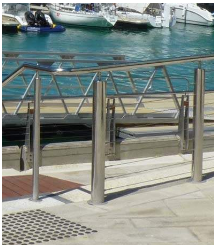
Stainless Steel balustrade with tensioned wire. Port Coogee, WA.
