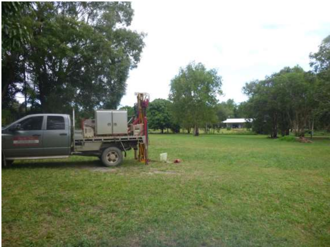
BH1 being drilled at 90 South Arm Drive, Wonga Beach.
