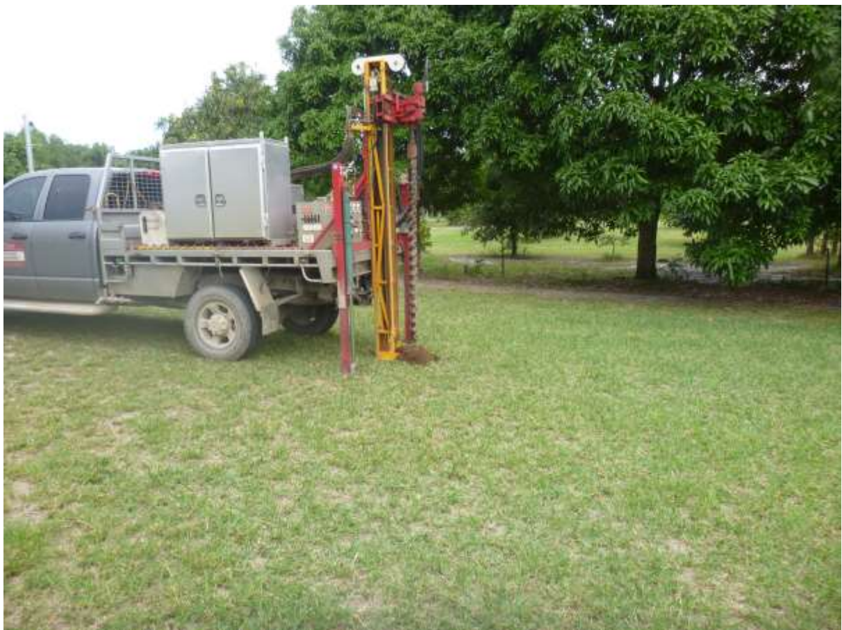
BH2 being drilled at 90 South Arm Drive, Wonga Beach.
