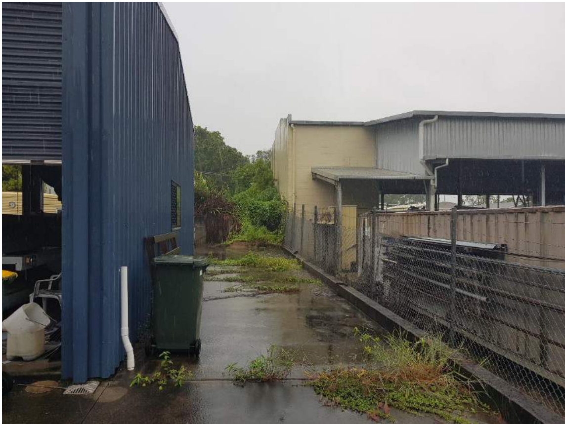
Side access to rear of the current building.
