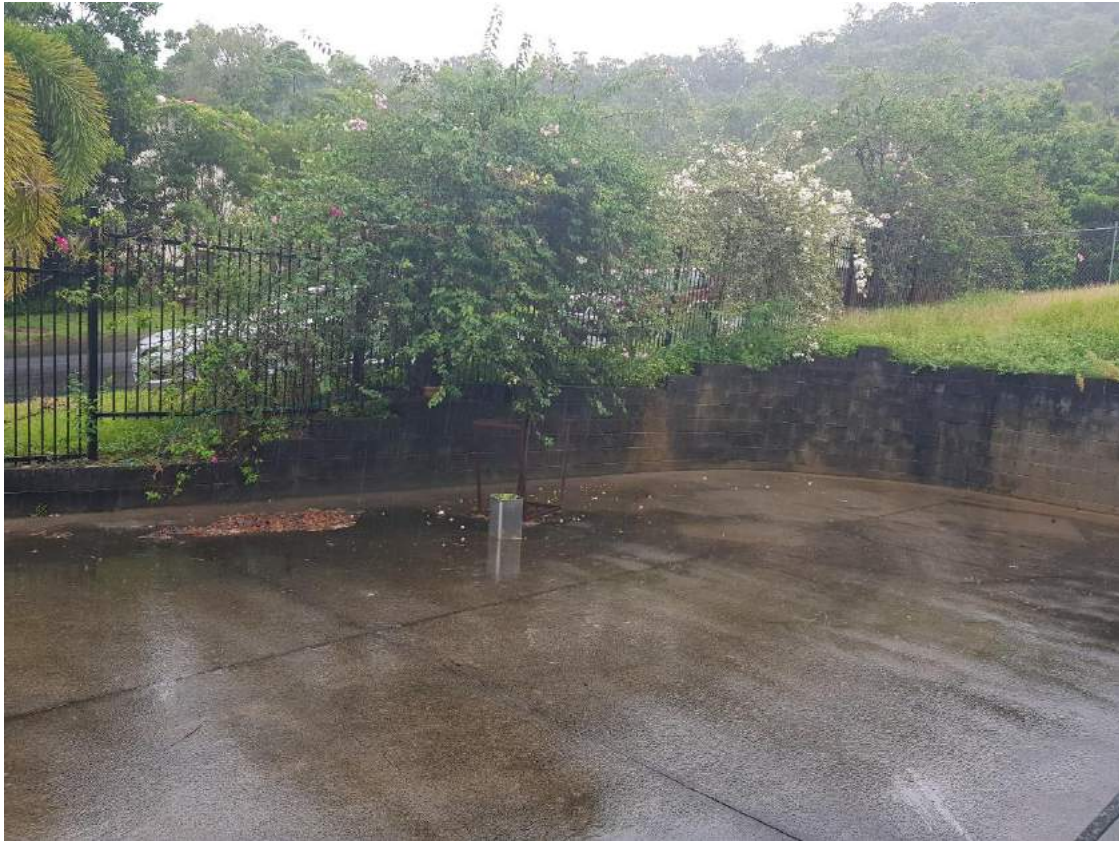
Current concreted area to be used as carparking. Some landscaping already established.
