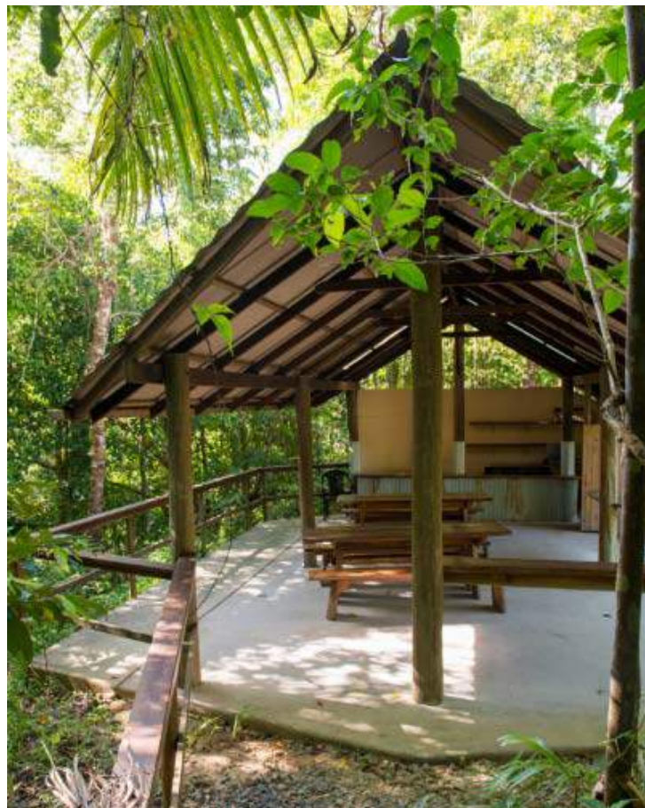
Photo 1 Existing Building Example -Design Style & Colour Scheme
