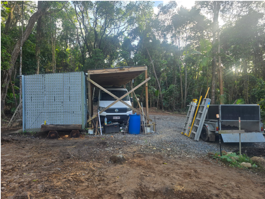
Figure 2: Existing sheds to be demolished.
