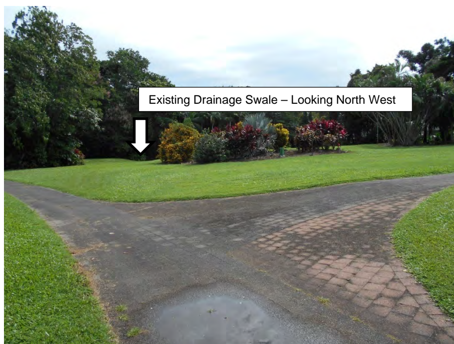
Photograph 6.1 – Existing Drainage Swale Directing Site Run-Off to Existing Outlet
