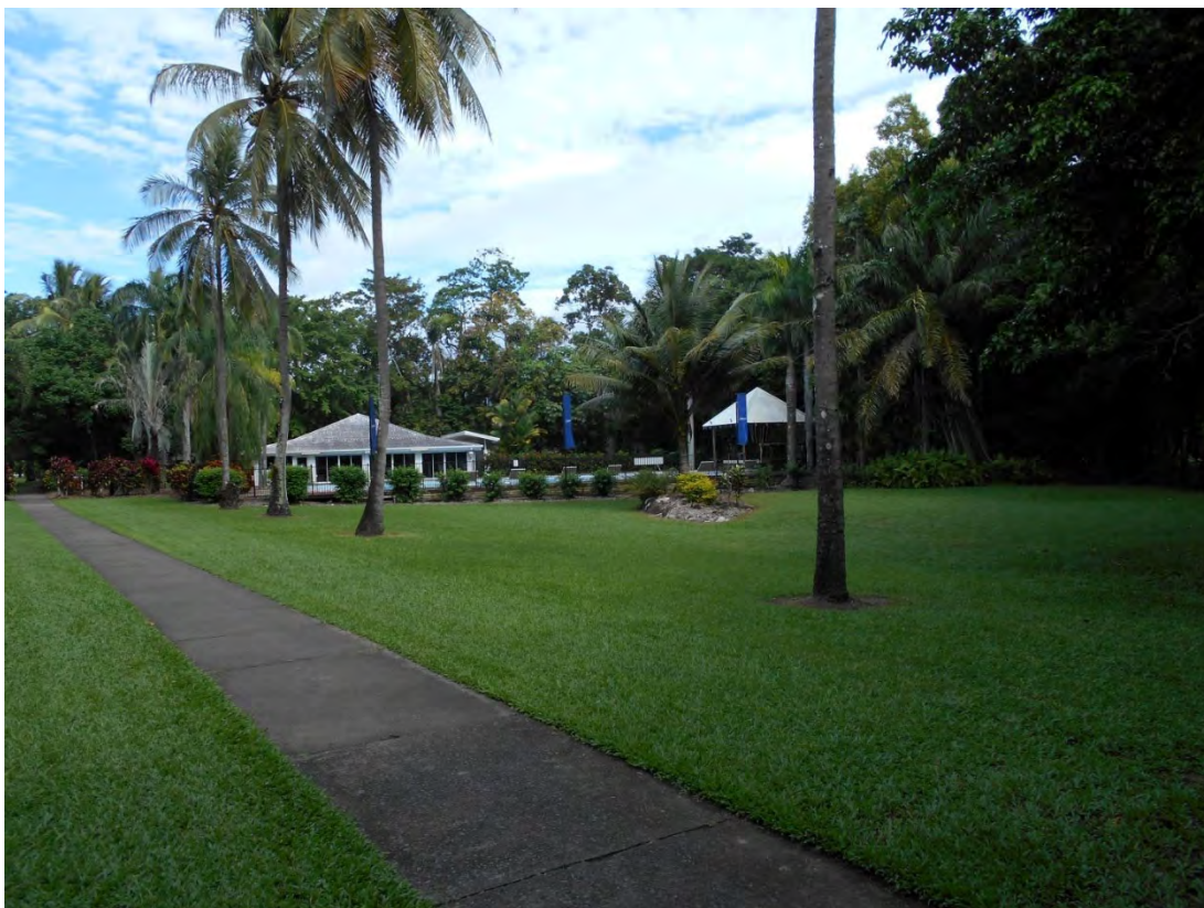
Photograph 2.1 – Existing Gymnasium and Pool from On-Street Pathway Looking South
