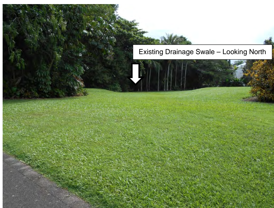
Photograph 6.2 – Existing Drainage Swale Directing Site Run-Off to Existing Outlet
