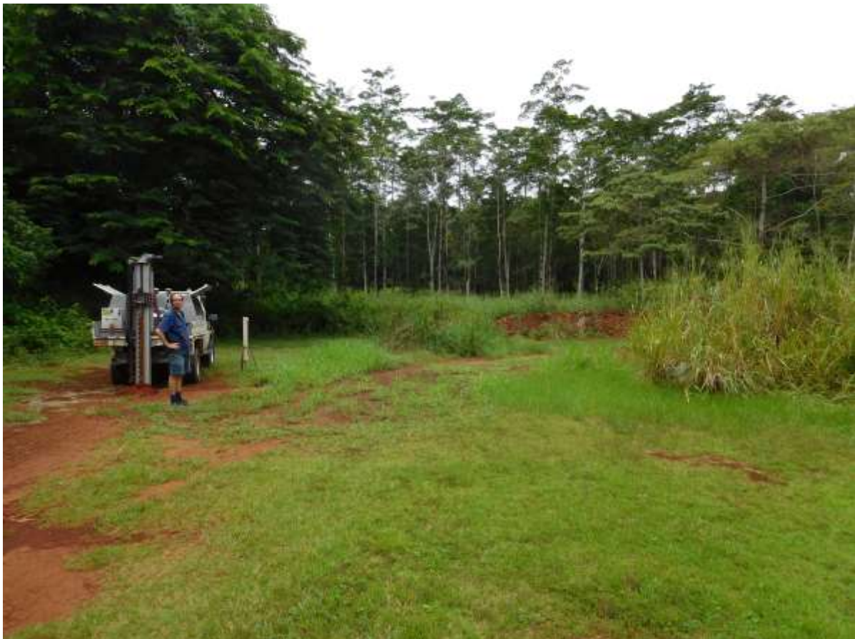
Permeability testing at 86 Ironbark Road, Diwan.
