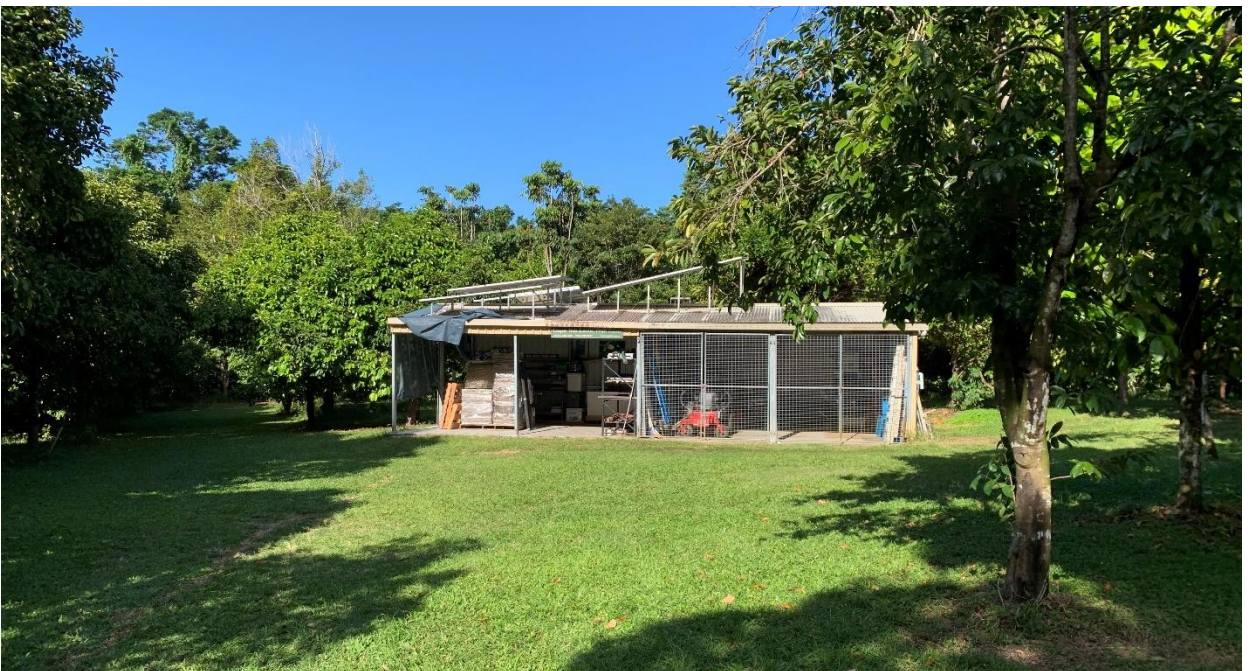
Photo 5: Existing Shed (Lot 4)
