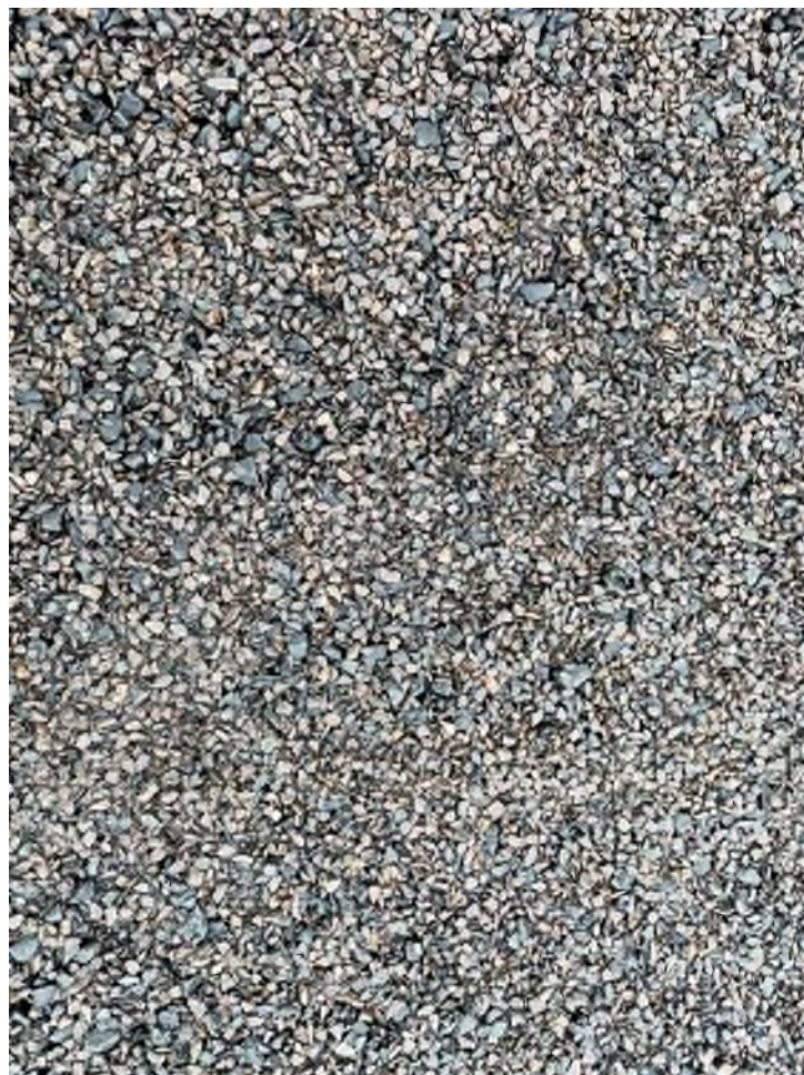
14/7 bitumen seal surface texture
