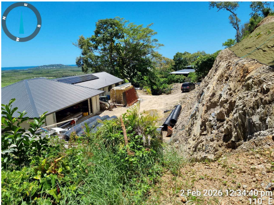
PHOTOGRAPH 5: View of Cut Batter behind Lot 14 dwelling (looking east)
