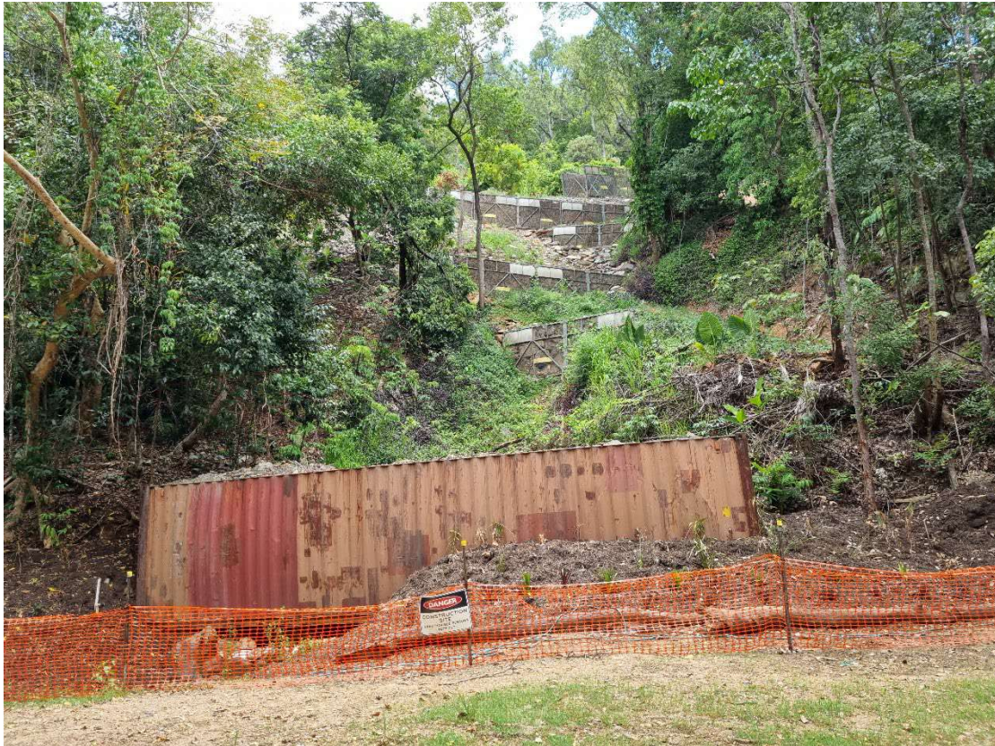
PHOTOGRAPH 2: View of Landslip Area after placement of cane bins (looking upslope from Ocean View Road)
