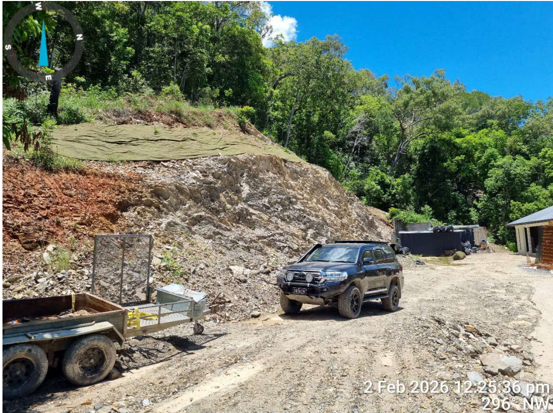
PHOTOGRAPH 4: View of Cut Batter behind Lot 14 dwelling (looking west)
