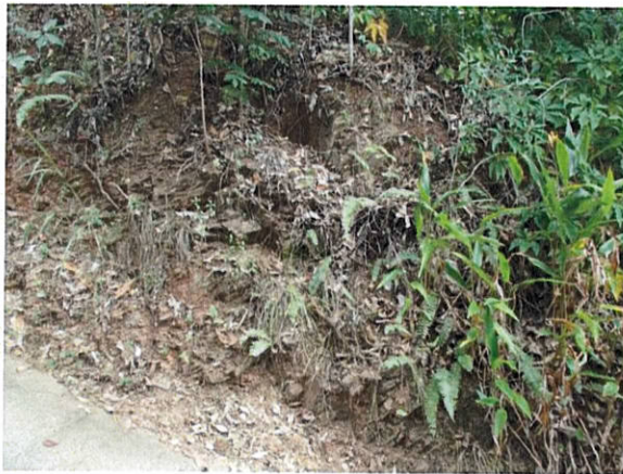
EXP10A: existing driveway cut batter (exposed rock at toe).
