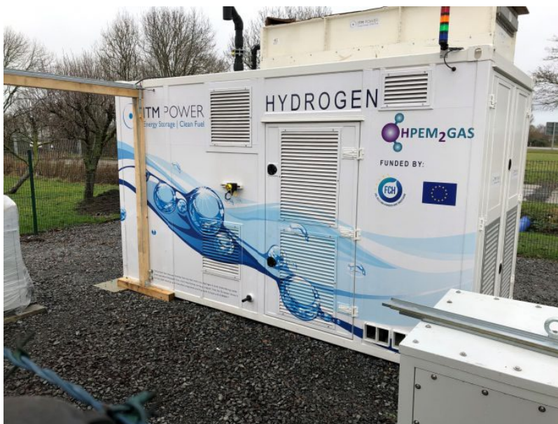
Figure 6 Typical containerised hydrogen electrolyser.
