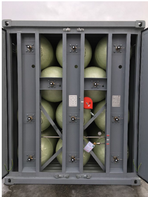
Figure 7 Typical low volume hydrogen storage.
