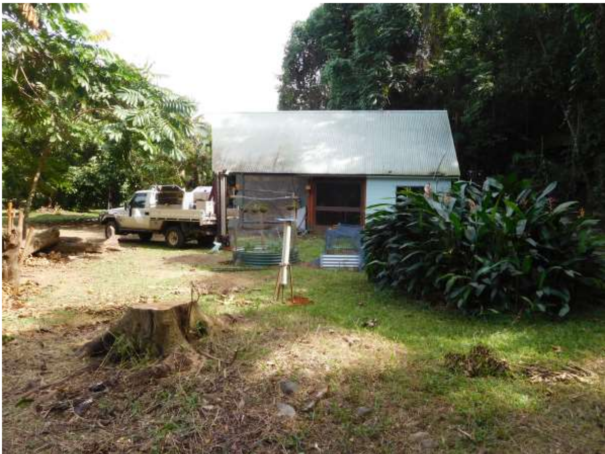
Permeability testing at 3939 Cape Tribulation Road, Cape Tribulation.
