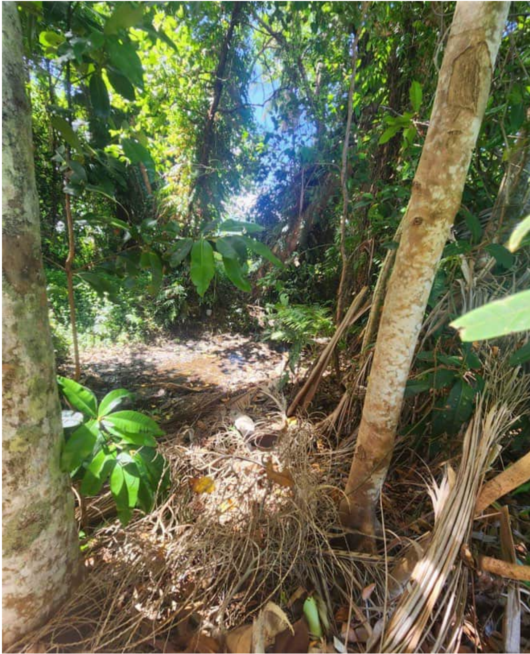
Figure 5 – Shallow drain which borders the unnamed road reserve which wraps around the western boundary of the site.
