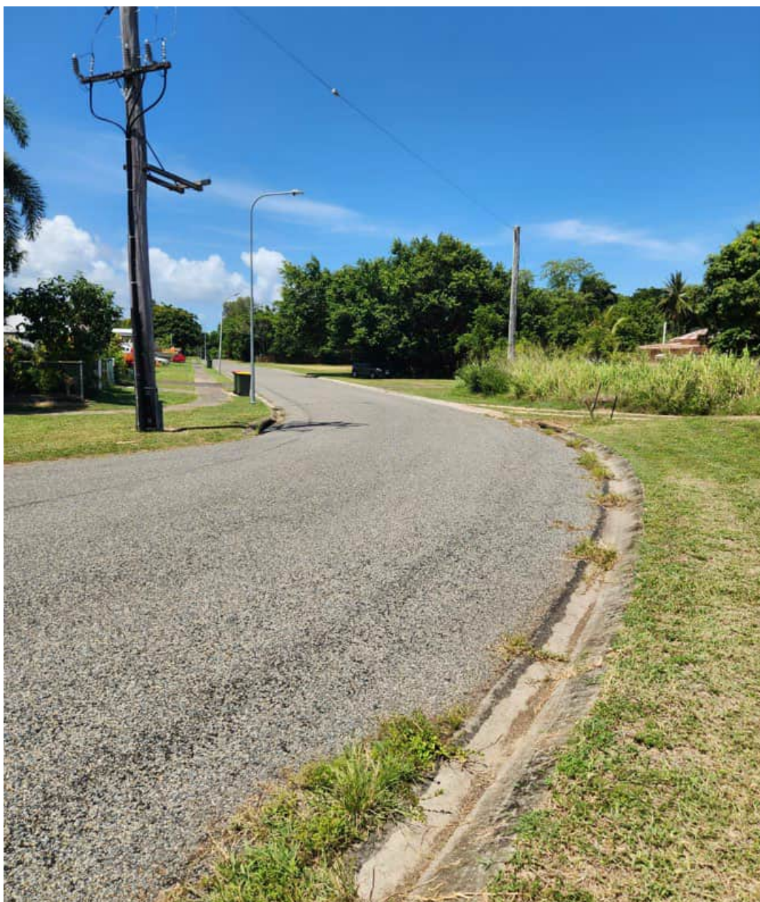
Figure 6 – Northern view from the site along Oasis Drive – note existing formed and sealed road, kerb and channel, footpath, electrical and lighting infrastructure.
