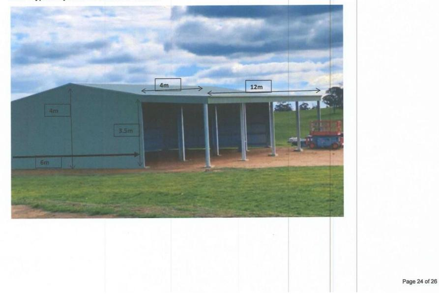
Shed Dimensions : 12m wide, depth 10m (including awning 4m depth), Height = 3.5m to gutter. Total 4m, Pitch 10o, Forest green or like.
