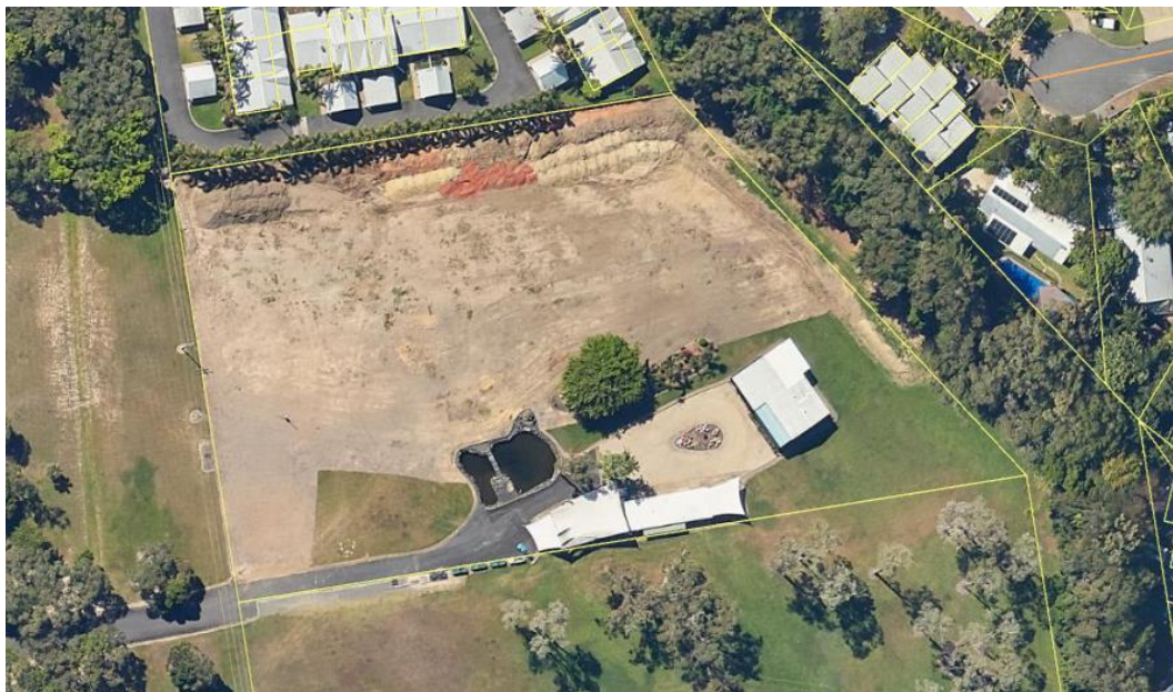
Image 2 Qld Globe August 2023 – spoil piles along northern boundary of site and appearing to extend east into drainage path lot
