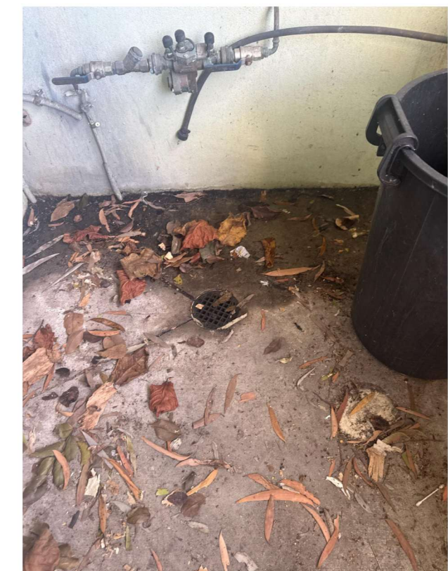
EXISTING WASHDOWN DRAIN
