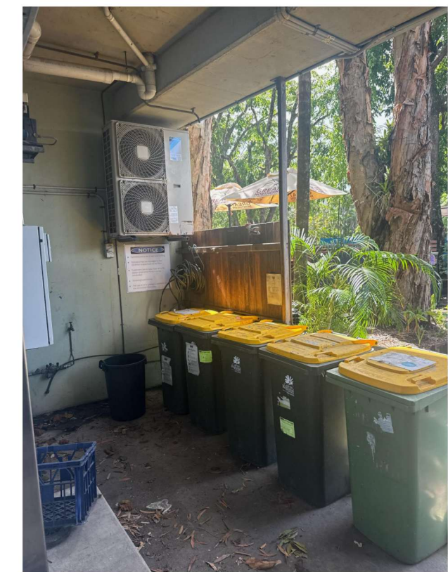
EXISTING WASHDOWN HOSE COCK
