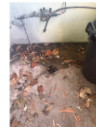
EXISTING WASHDOWN DRAIN
