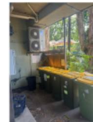
EXISTING WASHDOWN HOSE COCK
