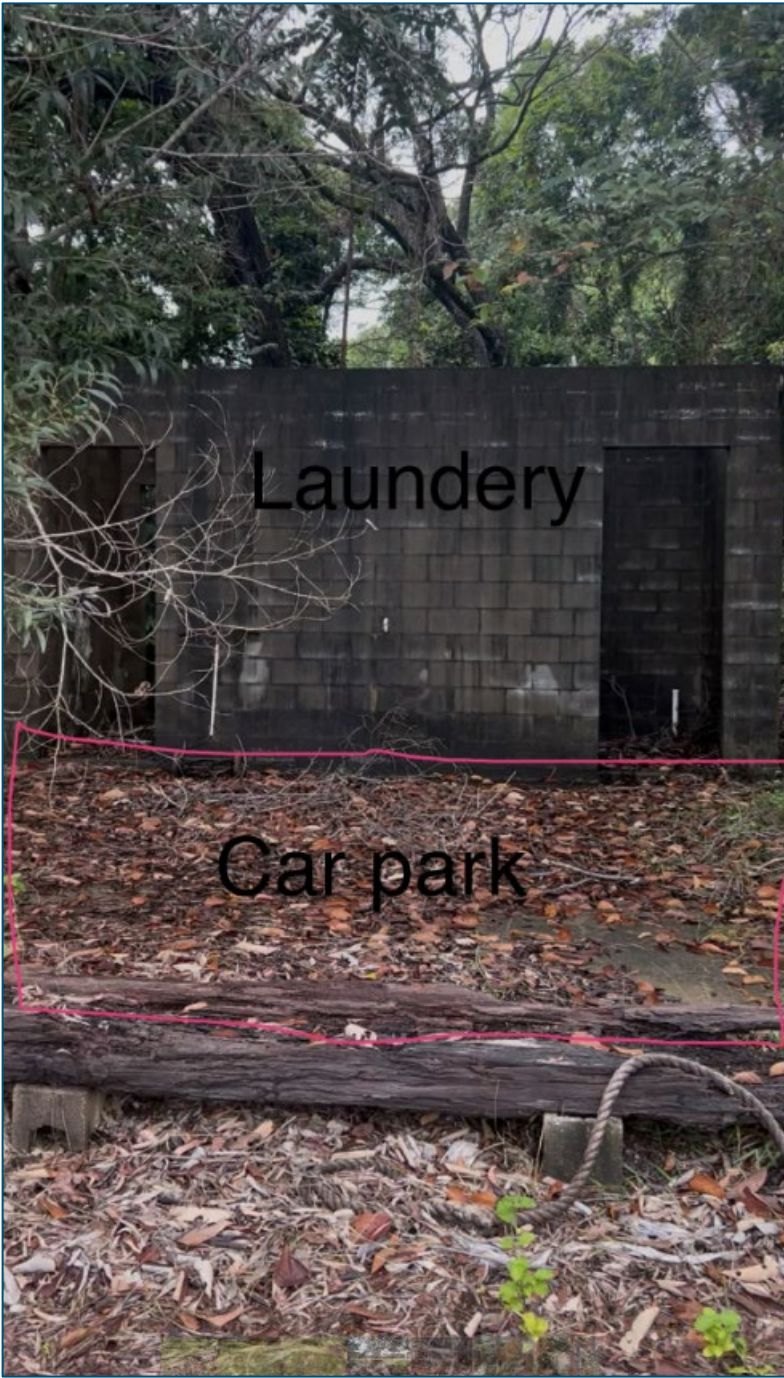
Photograph 3: Carpark Slab and Laundry (Source: Shell Engineers)
