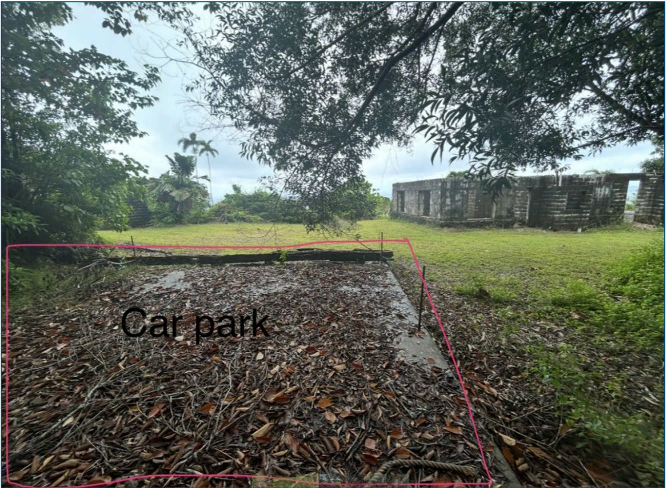
Photograph 2: Carpark Slab with Dwelling House in the background (Source: Shell Engineers)
