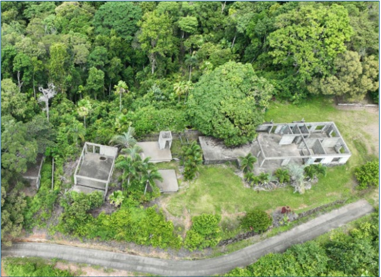
Photograph 1: Aerial View of Dwelling House and Home Based Business (3 x Bungalows) (Source: Shell Engineers)
