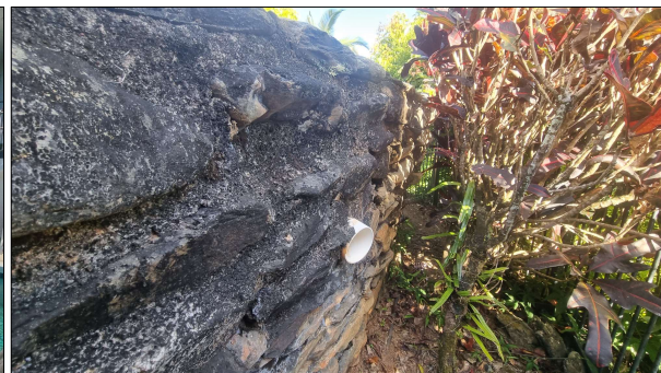
Figure 3: Retaining wall at northern boundary
