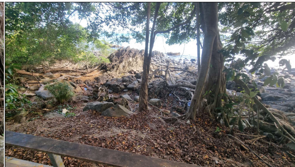
Figure 5: Bedrock present at base of slope
