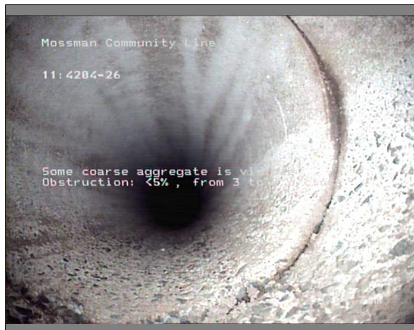
Photo: 11_12_53_A.JPG 1.76m, Some coarse aggregate is visible , Obstruction: <5% , from 3 to 9 o'clock
