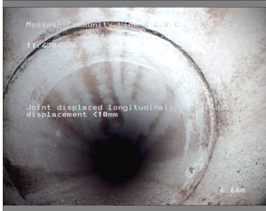
Photo: 11_12_54_A.JPG 6.66m, Joint displaced longitudinally, longitudinal displacement <10mm
