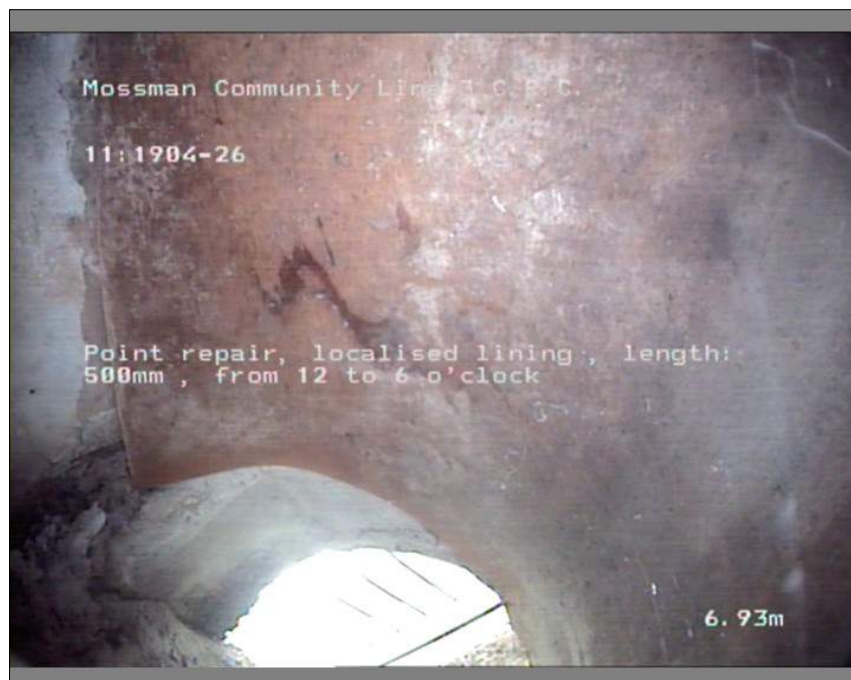
Photo: 9_10_43_A.JPG 6.93m, Point repair, localised lining, length: 500mm, from 12 to 6 o'clock
