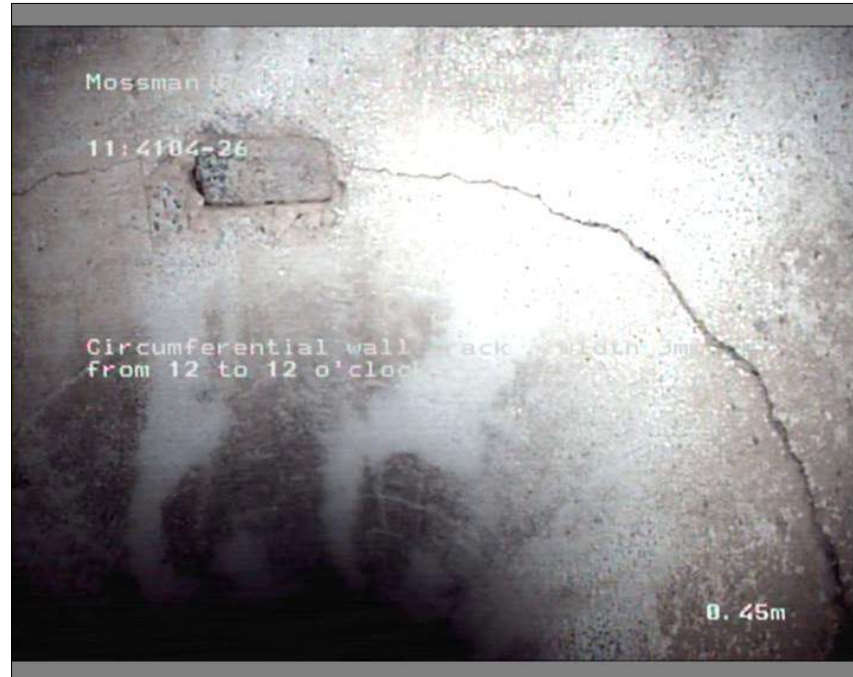
Photo: 11_12_52_A.JPG 0.45m, Circumferential wall crack , width 3mm , from 12 to 12 o'clock
