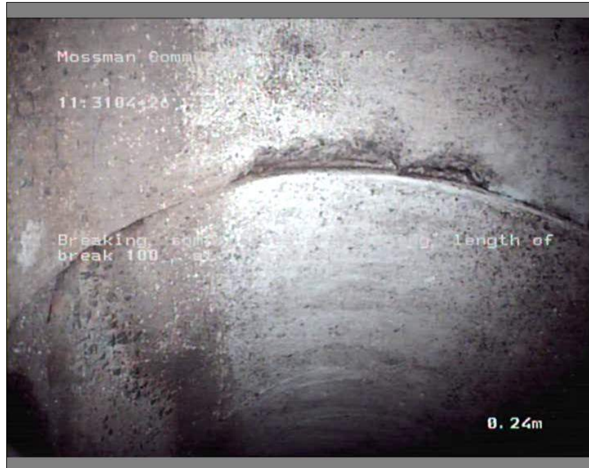
Photo: 10_11_47_A.JPG 0.24m, Breaking, some pieces are missing, length of break 100 , at 11 o'clock
