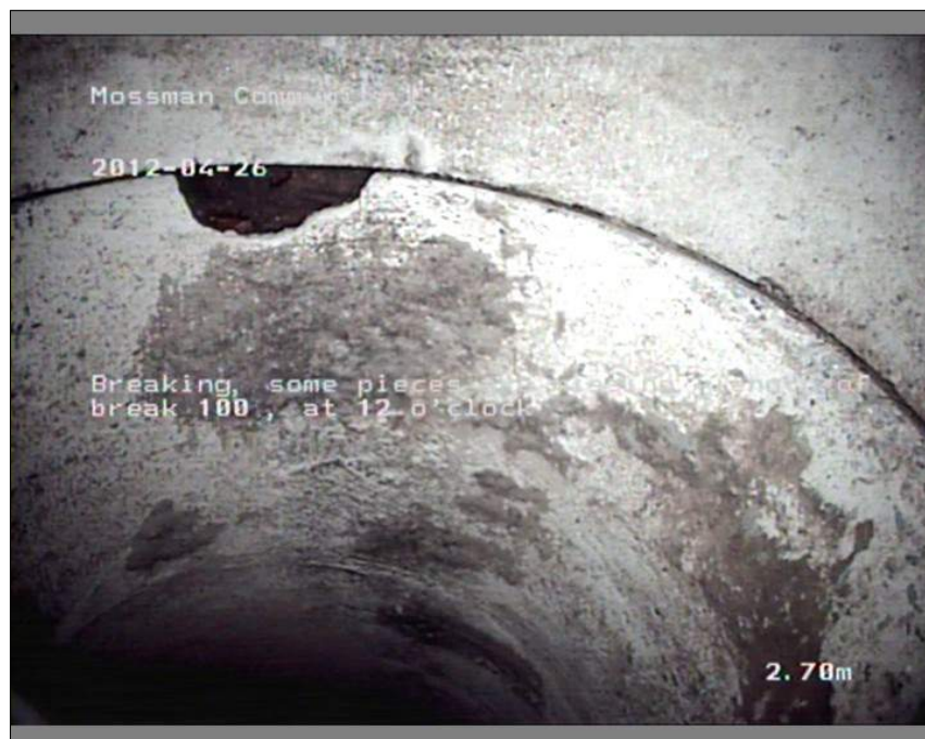
Photo: 10_11_48_A.JPG 2.7m, Breaking, some pieces are missing, length of break 100 , at 12 o'clock
