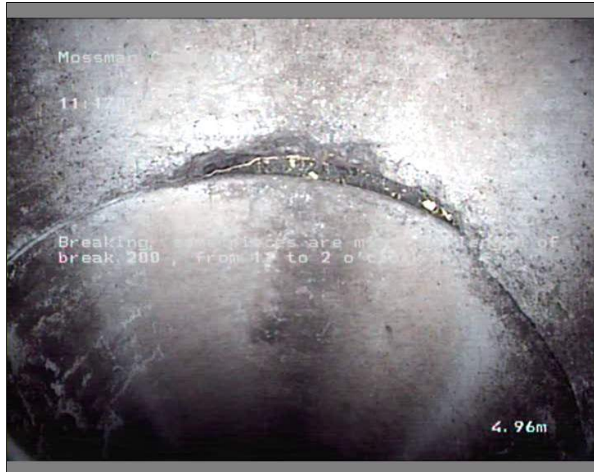
Photo: 9_10_42_A.JPG 4.96m, Breaking, some pieces are missing, length of break 200, from 11 to 2 o'clock
