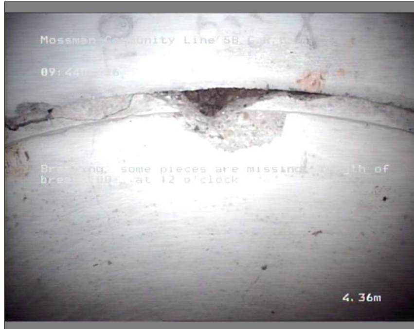
Photo: 5_6_20_A.JPG 4.36m, Breaking, some pieces are missing, length of break 100 , at 12 o'clock
