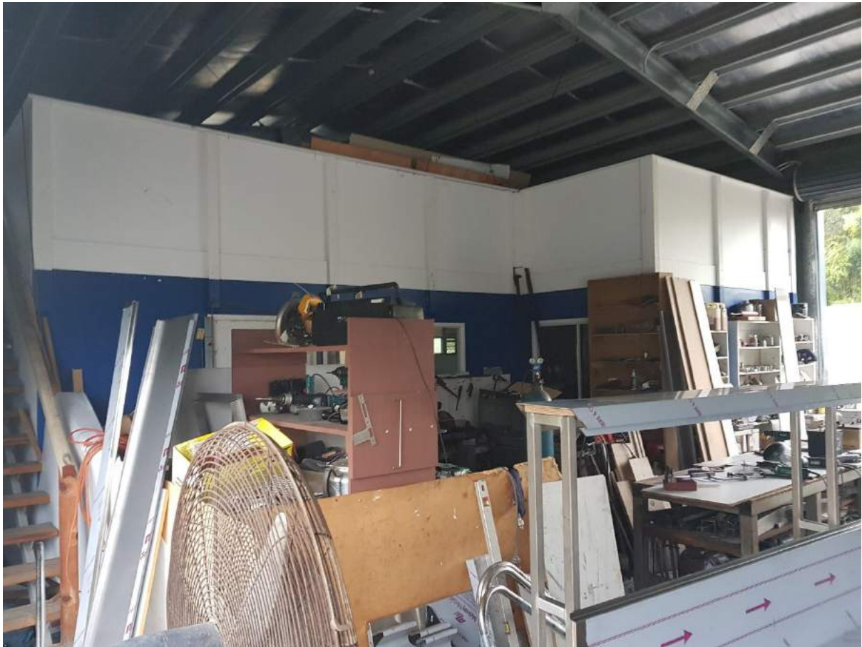
Image 1: Internal area and mezzanine.
