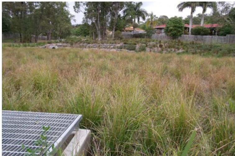
Figure 3 – Typical Bio-Retention Basin
