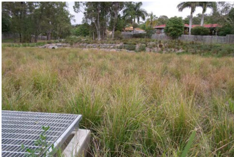
Figure 3 – Typical Bio-Retention Basin
