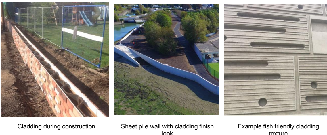
Figure 3-2: Sheet pile walls with textured capping beam or cladding 8 .
