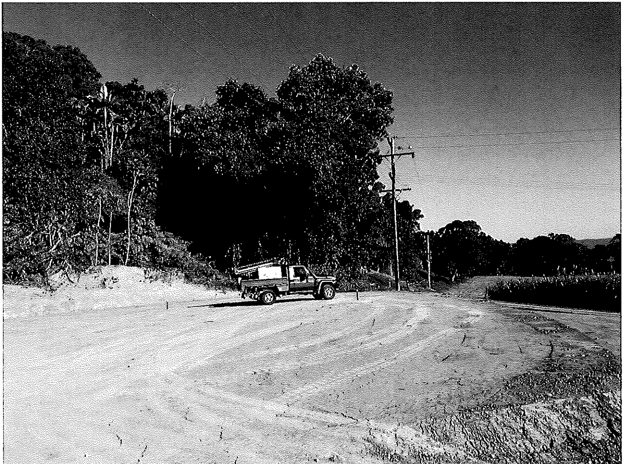
Site testing at Lot 3 Bamboo Creek Road, Miallo
