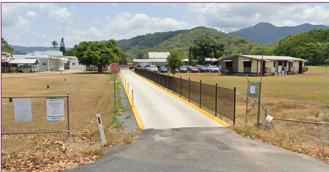
Figure 3: View from the Jack Street Frontage
