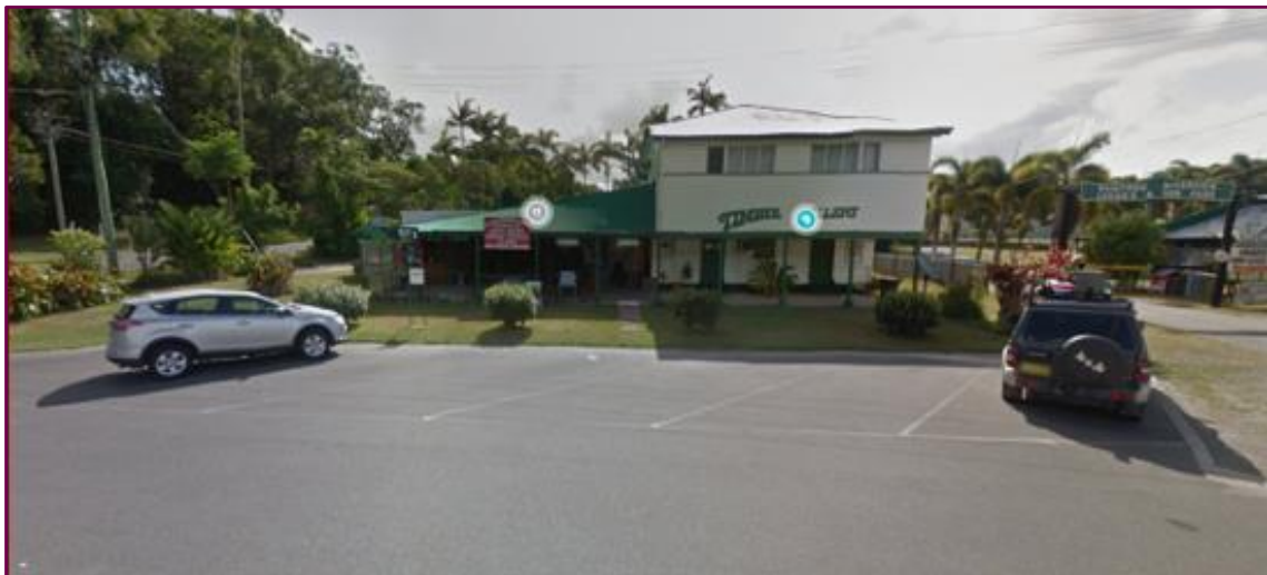
Figure 2 Stewart Street frontage
