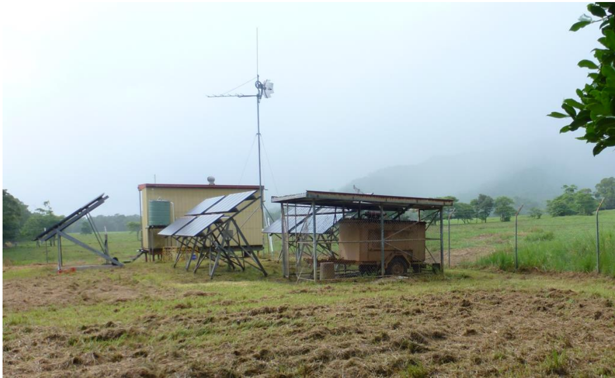
FIGURE 3 INTERNAL VIEW OF SUBJECT SITE SHOWING EXCHANGE SHELTER, SOLAR PANELS, GENERATOR AND 9M TRIAD
