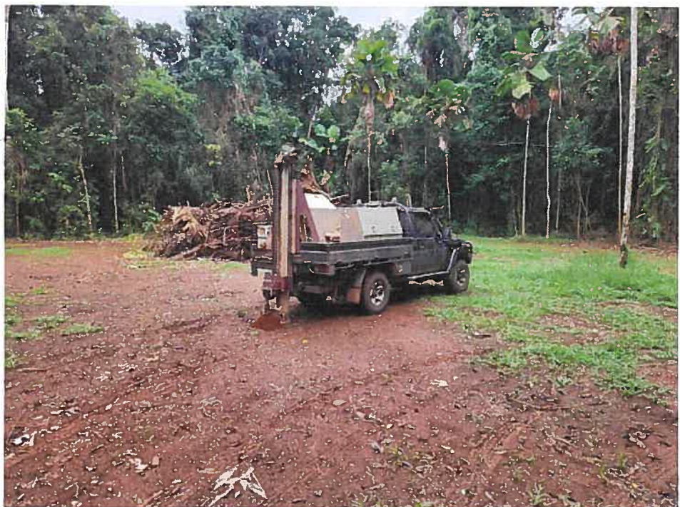
Site testing BH1 at Lot 7 Camelot Close, Cape Tribulation
