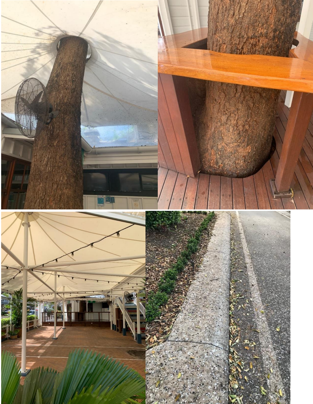
Above pictures are of Tree 88 and its trunk, its location to building and eating areas, and result of bird and bat droppings.
