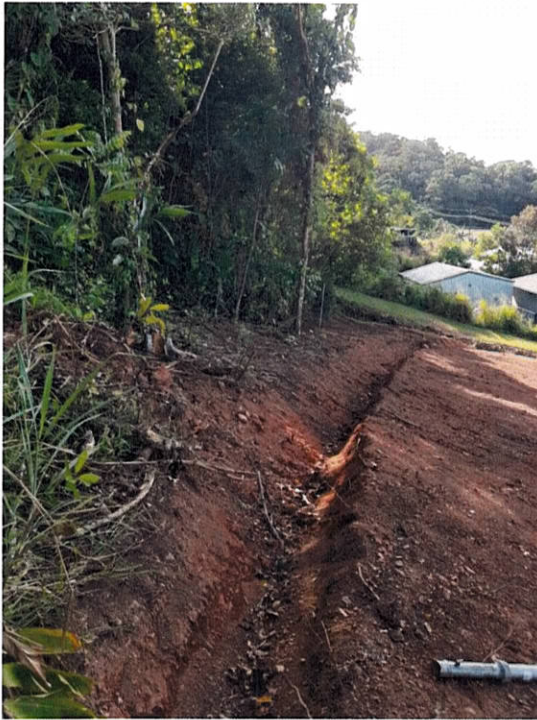
UPPER BATTER (BATTER No. 3) TOP DRAIN.
