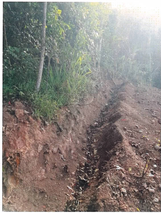
UPPER BATTER (BATTER No. 3) TOP DRAIN.
