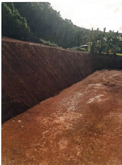
LOWER BENCH TO INTERMEDIATE BATTER (BATTER No.1).
