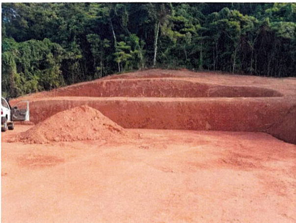
CONSTRUCTED SITE FROM LOWER BENCH to BATTER 1 to INTERMEDIATE BENCH to BATTER 2 to UPPER BENCH to BATTER 3 to NATURAL TOP SLOPE.
