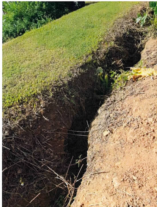
EXISTING RH DRAIN (deep scour).
