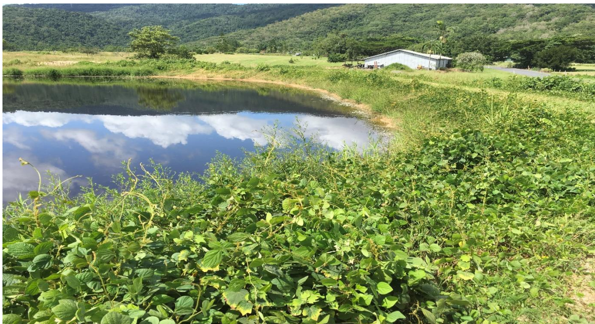
Photo of dam looking from east to west (towards Thomson Low Drive)
