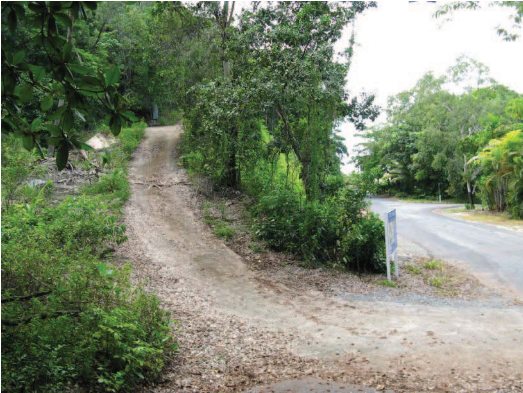
Plate 1 – View along sealed portion of existing service track, looking south-east
