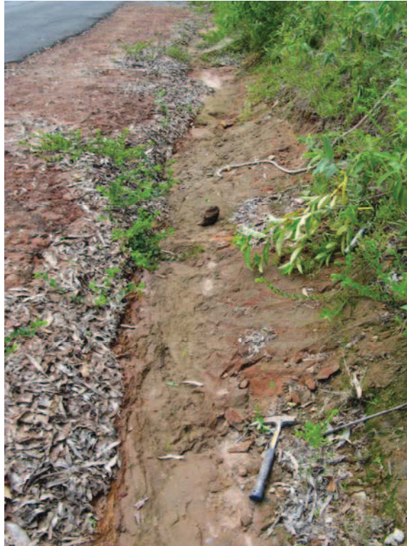
Plate 3 – View of bedrock in unlined stormwater drain at toe of cut
