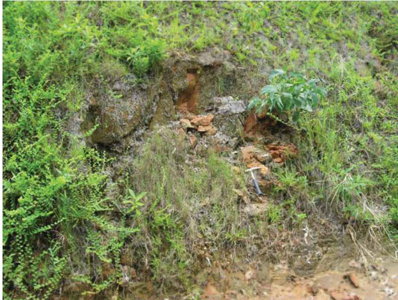
Plate 4 – View of small slope failure at toe of slope
