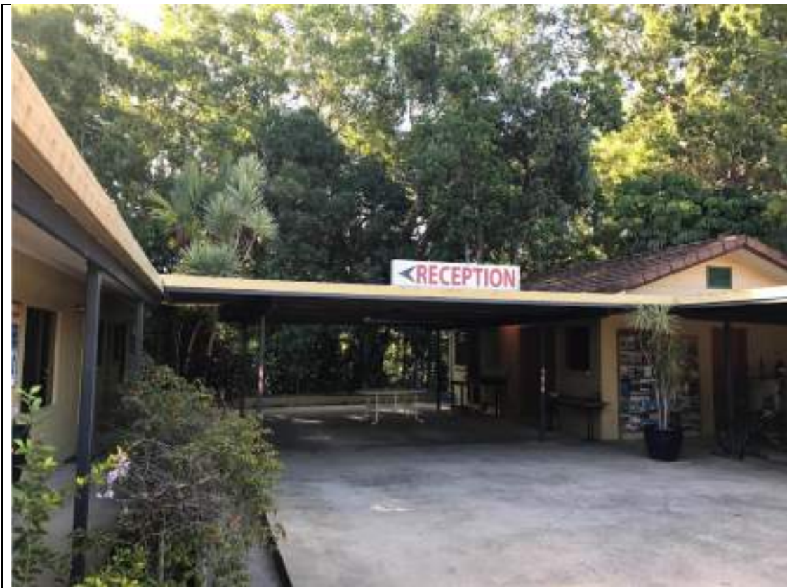
Photo 7: View west at the end of the internal driveway (managers unit and existing reception on left and laundry on right)
