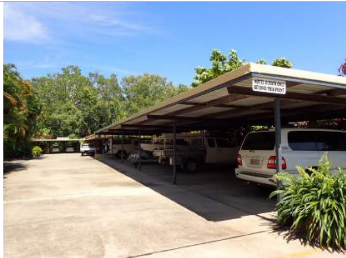
Photo 5: View west along internal driveway (awning structure to be removed)
