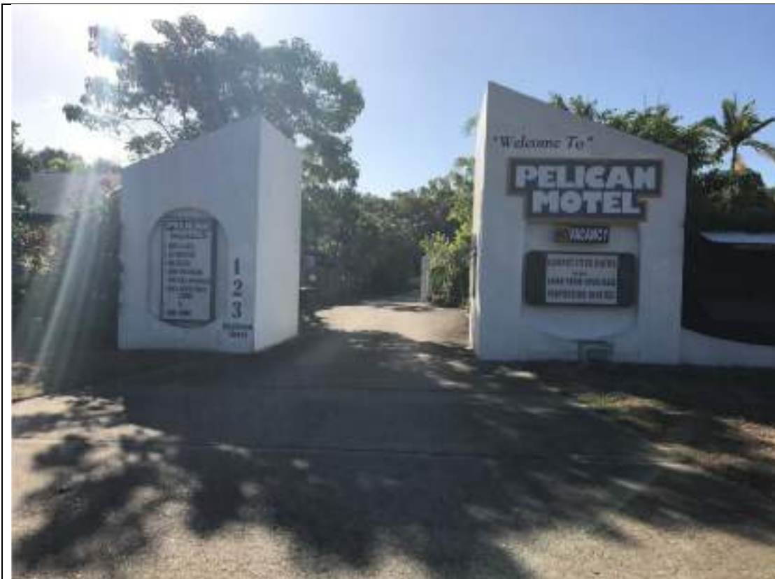
Photo 2: Front on view of site entrance from Davidson Street
